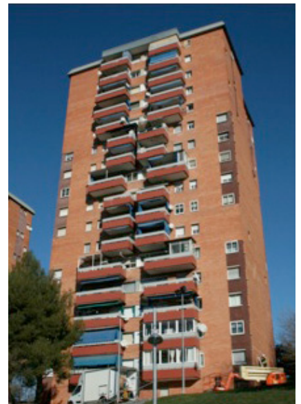
Energetic modernization: These existing apartment blocks in Spain will be insulated.
