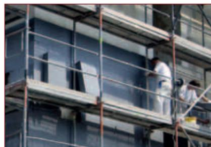
Facade insulation boards made of Neopor
