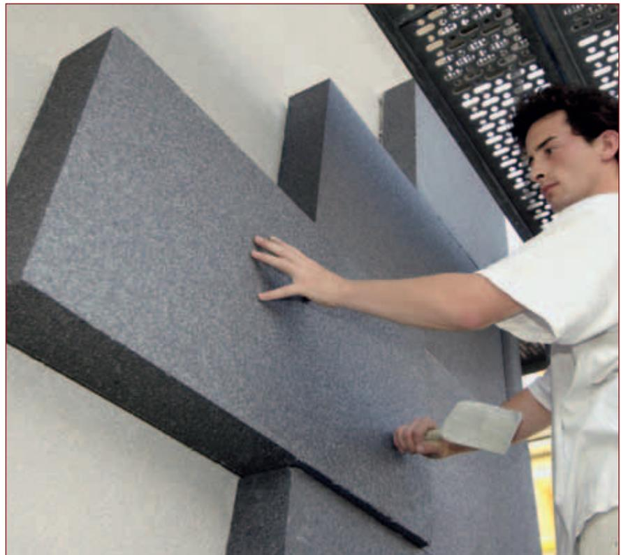
Secure adhesion of the insulation boards with sufficient adhesive according to the manufacturer's instructions
