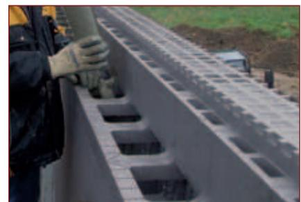
Insulating concrete forms (ICF) made of Neopor
