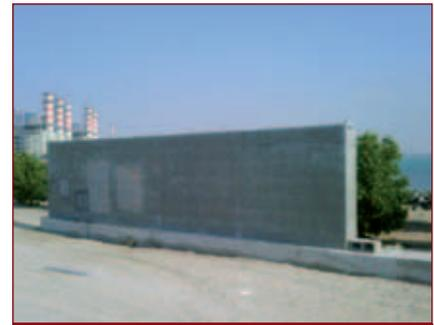
Test wall made of Neopor in Abu Dhabi
