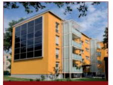
Zero-heating-energy house, Germany In order for the building to achieve the lowest possible heating costs, an external thermal insulation composite system with insulating boards made of Neopor was used. Energy for electrical power, hot water, and heating is obtained by using regenerative energy sources.
