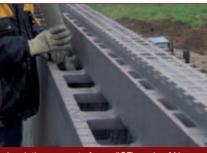
Insulating concrete forms (ICF) made of Neopo
