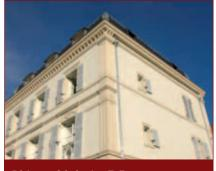
Bâtiment Génération E, France Complete renovation of an old town house villa near Paris. Reduced energy consumption from 400 kWh to less than 50 kWh per m<sup>2</sup> is obtained primarily by insulating the exterior walls (ETICS), the roof, the floor, and ceilings with Neopor<sup>®</sup>.
